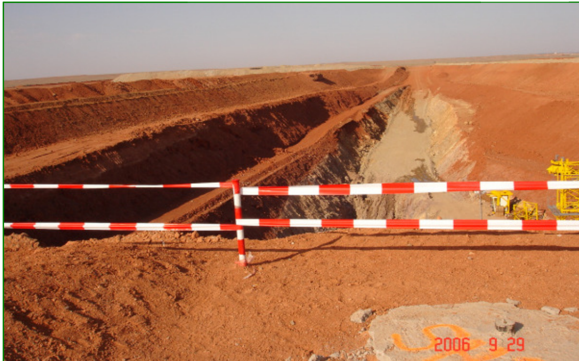
Photo 1. Preparation work for Shaft #2 on OTD 1259
