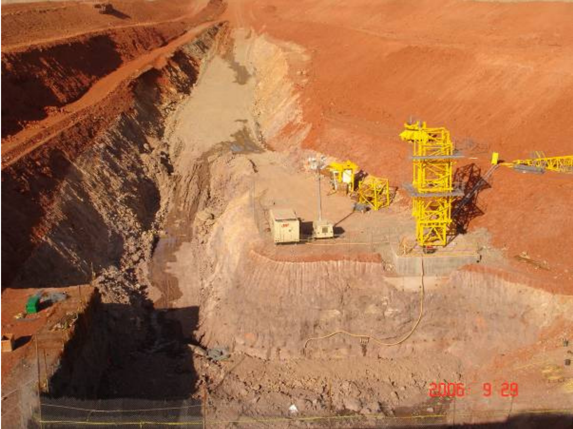
Photo 2. Main technological operation during the shaft sinking
