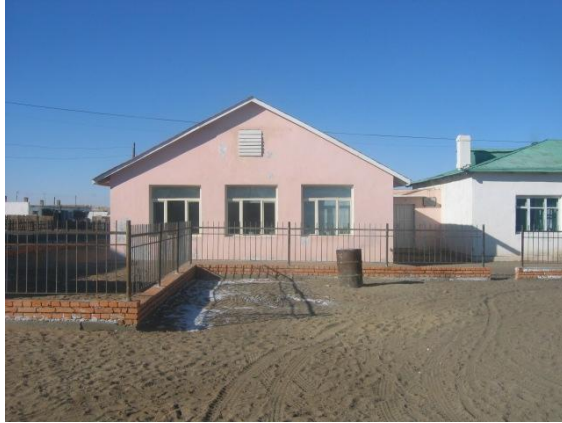
Kindergarten yard is improved and built fence.
