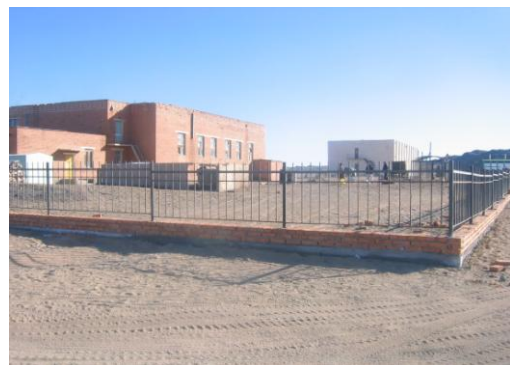
New fence erected for the school.
