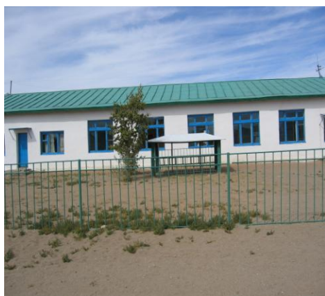
Khanbogd hospital façade, 2004
