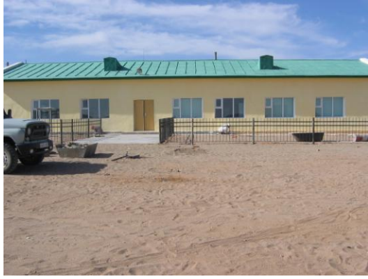
Khanbogd hospital façade, 2005.
